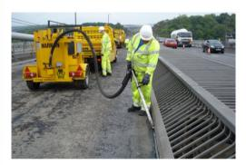
Phoenixsed!® SH10 is another type of fine polymeric hot applied mastic that is especially designed for expansion joints on bridges.
