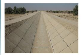
Hight elasticity, excellent adhesion to concrete surfaces and tolerance for different atmospheric conditions and thermal changes are among the characteristics of **Phoenixsed SH20**. Furthermore, this product is perfectly stable in the slopes of trapezoidal canals and would not slide down as time goes by.
